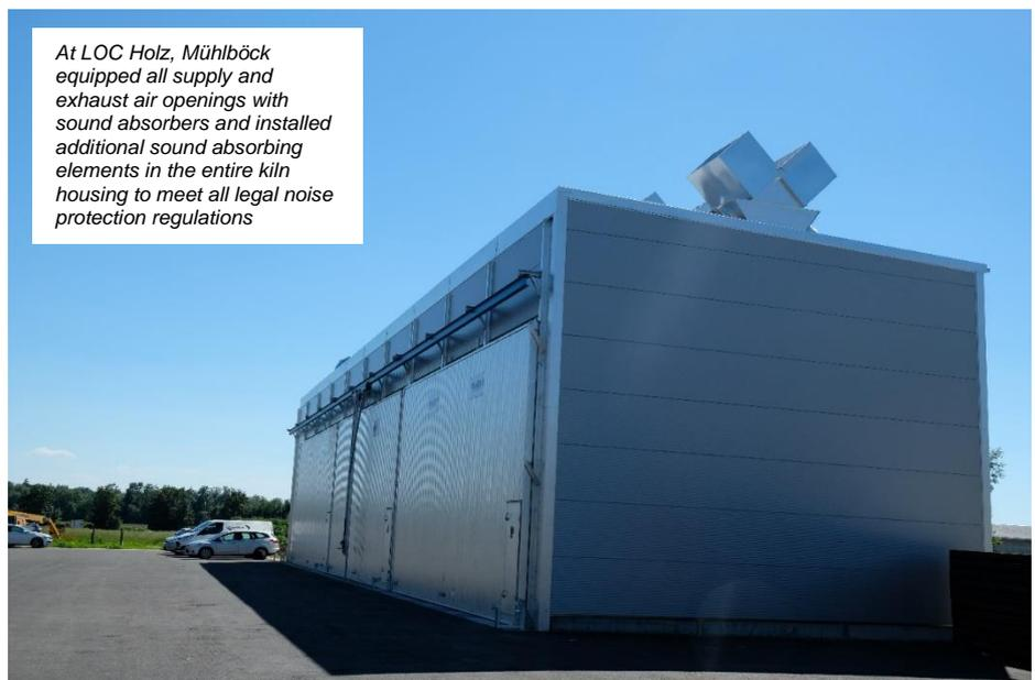
*At LOC Holz, Mühlböck equipped all supply and exhaust air openings with sound absorbers and installed additional sound absorbing elements in the entire kiln housing to meet all legal noise protection regulations*
